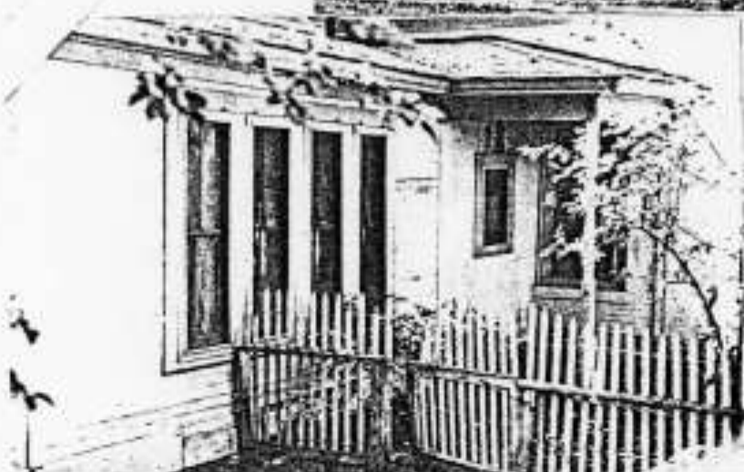
East back porch which been closed in to form a bath and a small room & half-bath South wall of east bedroom is shown at right
